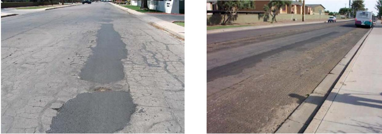
**FIGURE 1 (a) Pavement Section before the Fiber-Reinforced Asphalt Concrete Mixture Overlay; (b) Surface Preparation by Milling off the Edge of the Pavement.**
